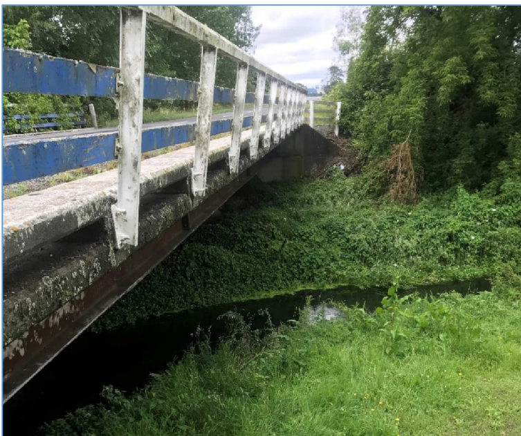
Figure 2.2: Kahahakuri Stream Bridge on Ongaonga Road
